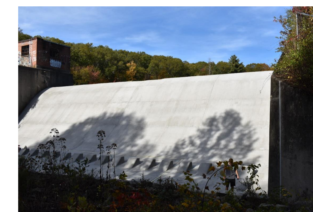
Figure 5: This wall is what guides the water as it runs out of the reservoir when it overflows. The water runs down this white platform into the brook.
